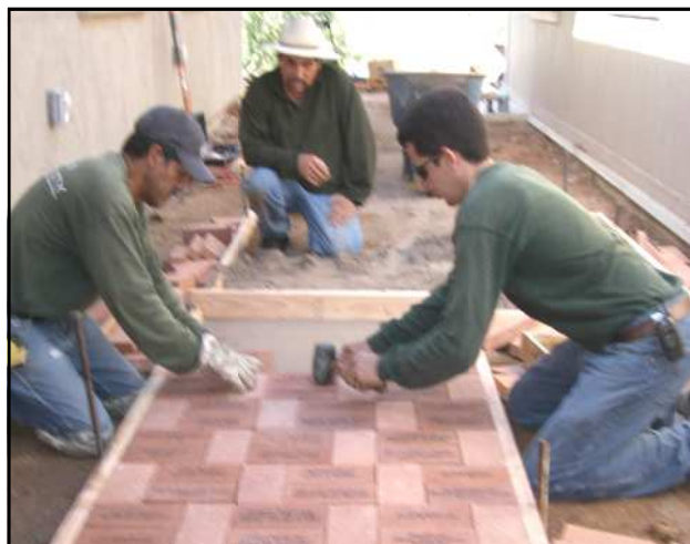
Garden of Caring — Workers from La Cholla Landscaping lay inscribed bricks to create the Garden of Caring between the old and new wings at ICS. Our thanks also to volunteers Earl White, Terry Watson and Tim Powell , who built a small garden outside the Food Bank entrance.
